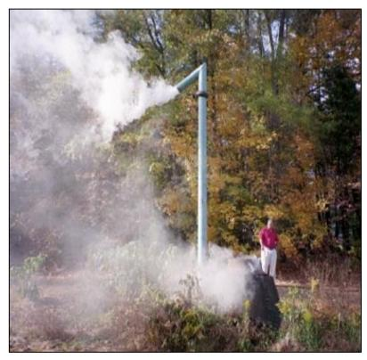
Figure 7-4 Uncontrolled Air Release Caused by Hydraulic Surge
