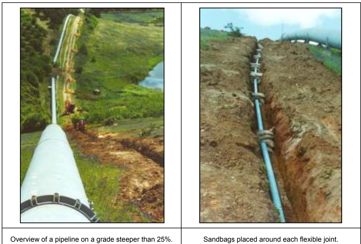
Figure 7.2 Pipe Anchorage on Grades Steeper than 25%.
